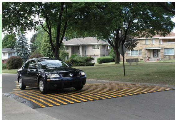
Gambar 2 2 Model Speed Table (trafficlogix)
